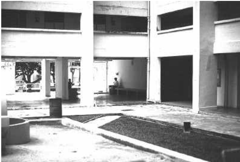
Figure 8: A Void Deck
